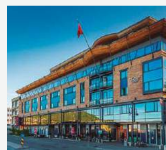
Thon Hotel Harstad. Hotel. Harstad, Norway. PACi, VRF and Refrigeration.
